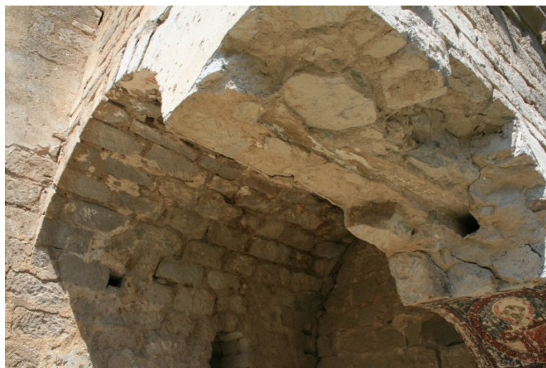
Fig. 14: St. George church (Karagedik Kilise), Peristremma (Belisırma), Cappadocia, cavities left in the place of notched wooden reinforcements at the springing of the vault in the NE corner (July 2009)
