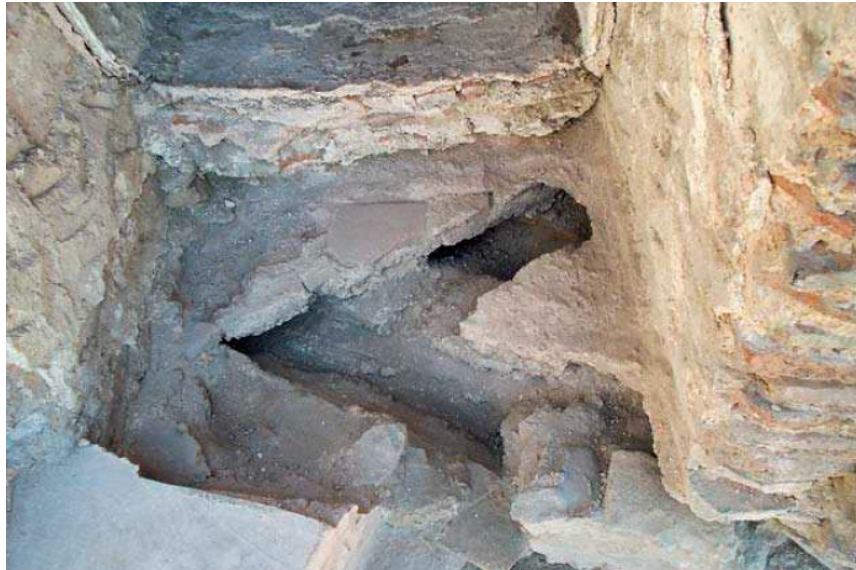
Fig. 16: Christ Pantocrator chapel (Zeyrek Camii), Istanbul, window reveal of the west central dome, showing the cavities for reinforcement beams at its base (July2003) (Ousterhout et al 2010, Fig. 7)
