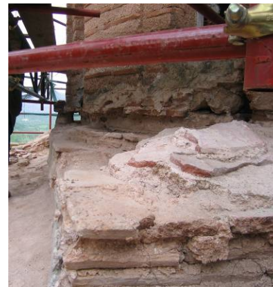
fig. 20 Panagia Krina, Chios, exterior view showing the position of wooden reinforcements at the base of the dome drum (Vintzilaiou 2006)
