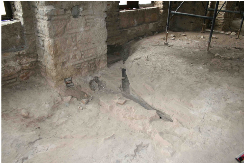
Fig. 50: Panagia Parigoritissa, Arta, cavities of wooden reinforcements in the dome vaults of the gallery (March 2007)
