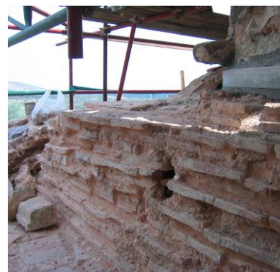
fig. 20 Panagia Krina, Chios, exterior view showing the position of wooden reinforcements at the base of the dome drum (Vintzilaiou 2006)
