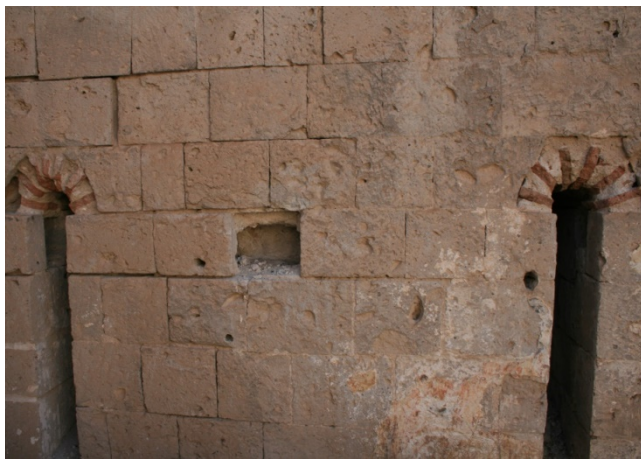
Fig. 40: Çanlı Kilise, Aksaray, Cappadocia, continuous wooden reinforcement at the springing of the main window arches, interior looking north (July 2009)
