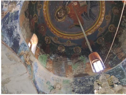
Fig. 25: St. Mary, Kosinë, Albania, view of wooden reinforcement ring at the base of the drum on the interior (September 2014)
